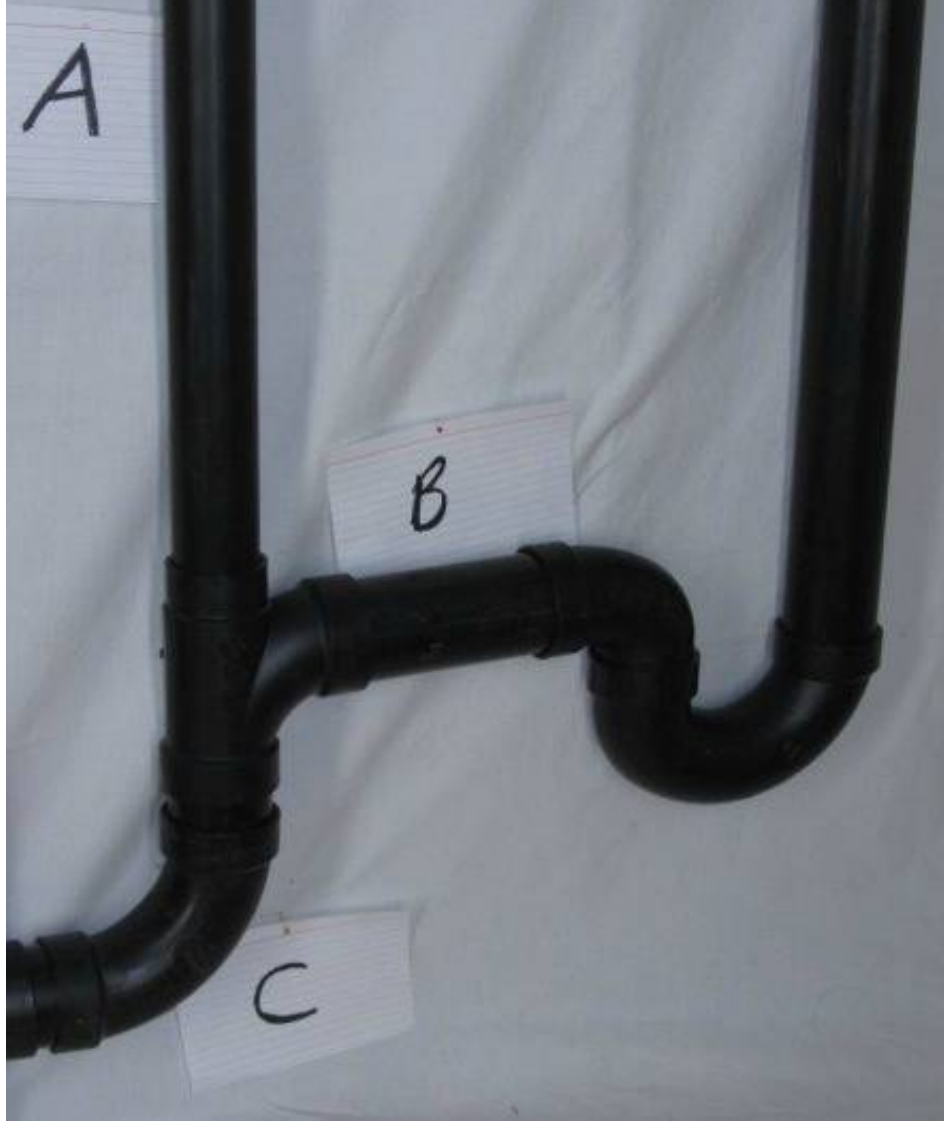
Installing A Washer Standpipe
